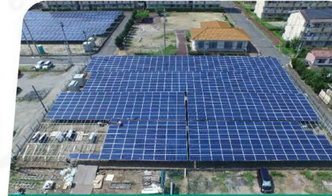
Project size: 700KW Site Location: Japan Finished Time: 2015 Project type: ST1 Steel Ground Mounting
