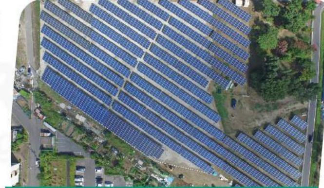
Project size: 1MW Site Location: Japan Finished Time: 2015 Project type: ST1 Steel Ground Mounting
