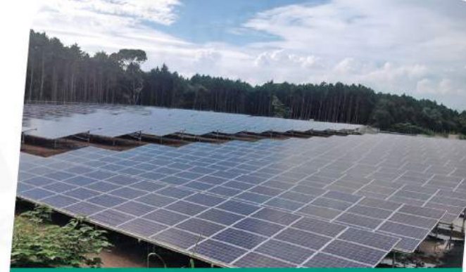
Project size: 7MW Site Location: Japan Finished Time: 2014 Project type: ST3 Aluminum Ground Mounting
