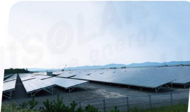
Project size: 30MW Site Location: Netherland Finished Time: 2017 Project type: ST3F Aluminum Ground Mounting
